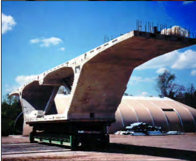
BRIDGE SECTIONS CAST ON SITE
