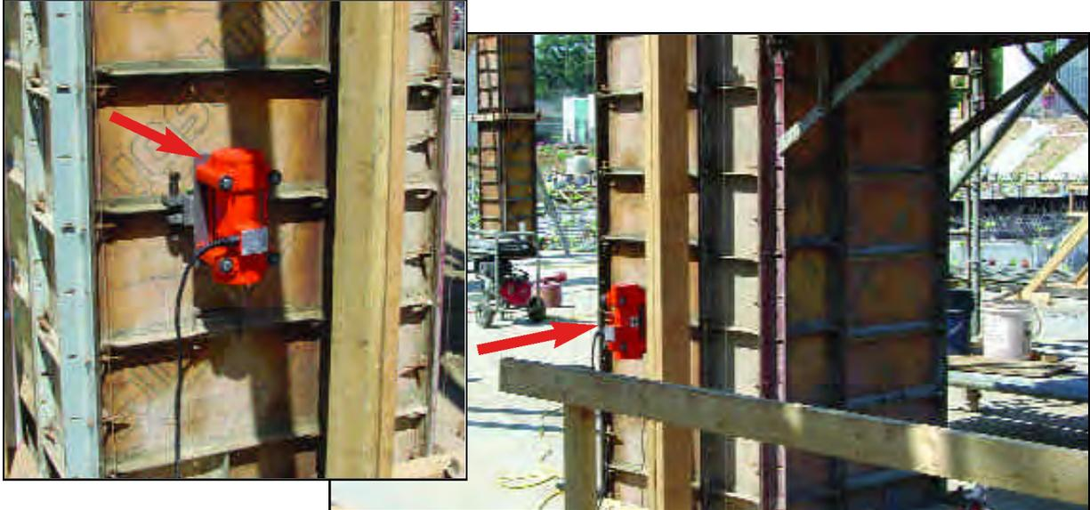
**PROBLEM:** To ensure placement of dense concrete with architectural finish in 24" square x 28 foot tall supporting piers.
