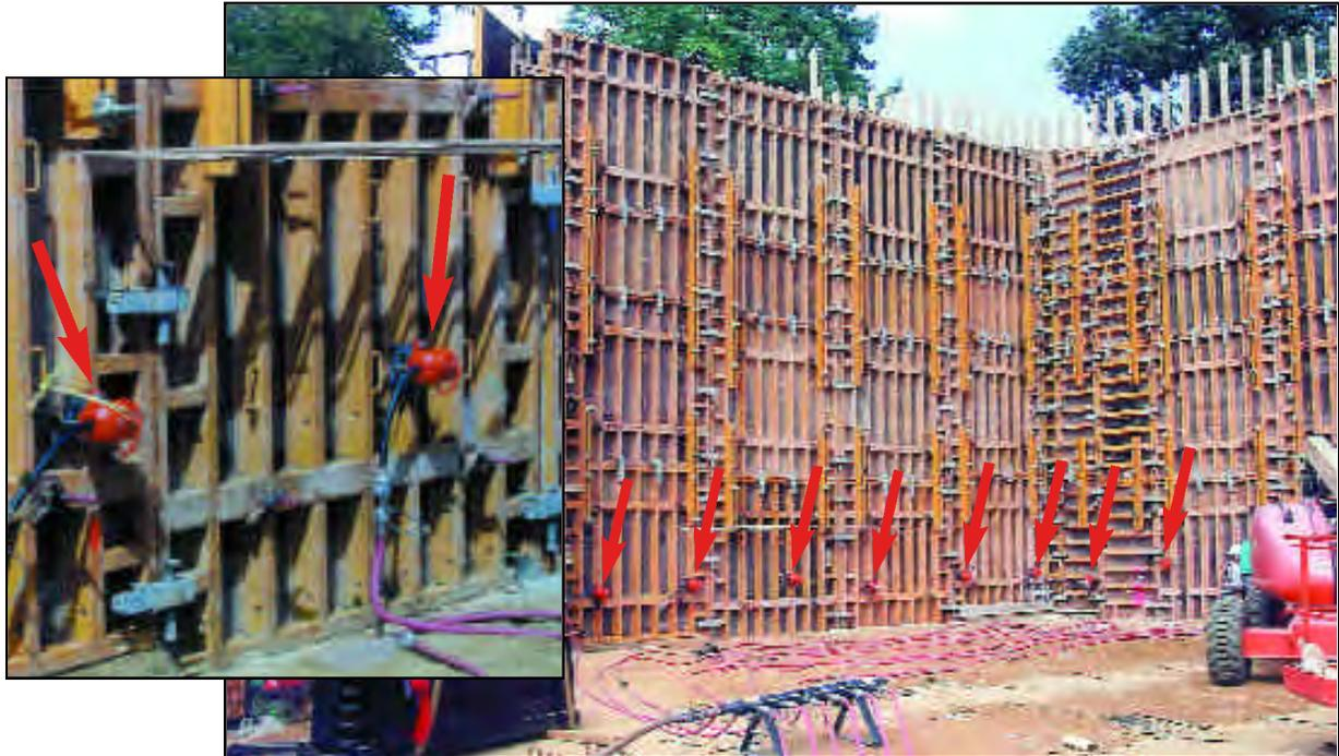
**PROBLEM:** A contractor had a very tall wall where the exposed side had to be blemish free. The rebar spacing was very tight, so it was almost impossible to get an internal vibrator down inside the wall form.
