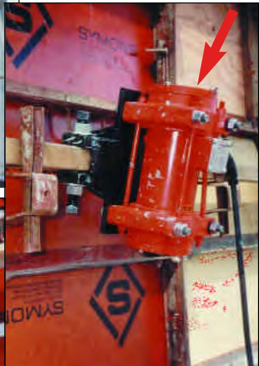
Bracket with vibrator clamped to a 2 x 6.
